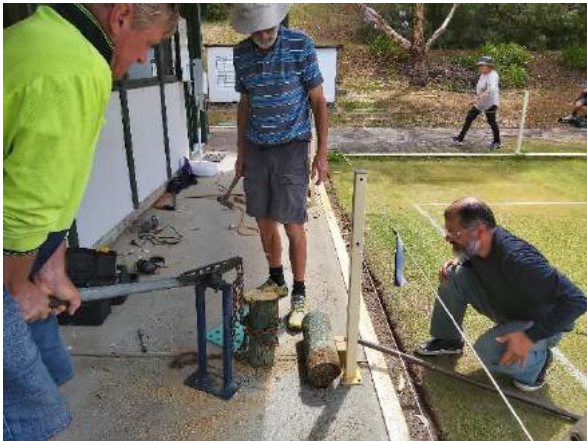
Removal of poles
