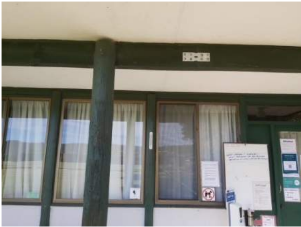
Preparation Work - Brackets installed, and extra supports added in the ceiling area
