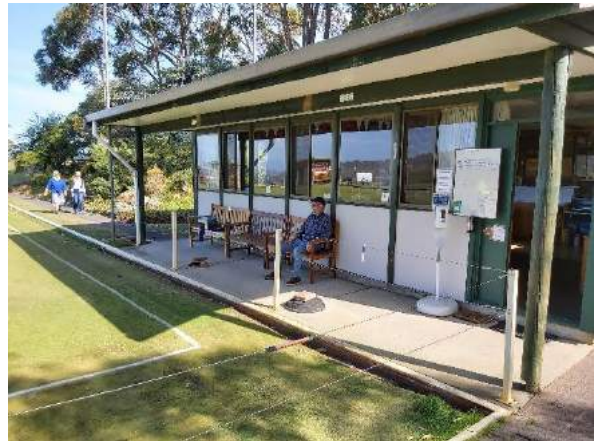
The clubhouse without central poles
