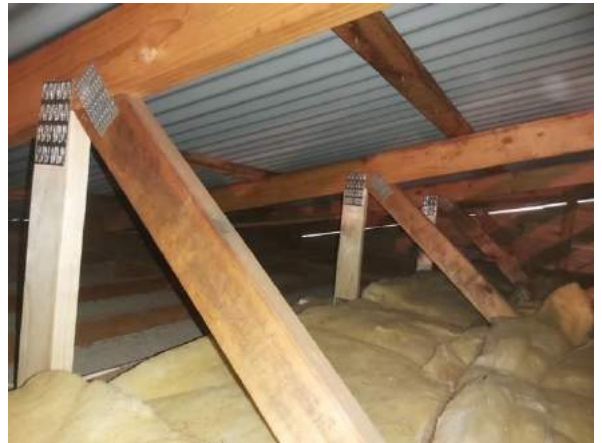
Preparation Work - Brackets installed, and extra supports added in the ceiling area
